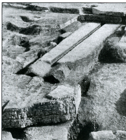
Granite cable channel excavated beneath the floor of the funerary temple of Chephren in 1909.
