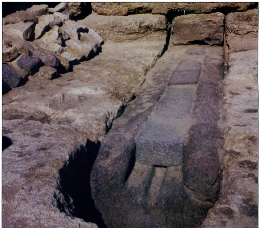
Cable channel carved into bedrock beneath the Sphinx Temple. It is plugged with a granite slab estimated at around 100 tons; the slab has a central groove filled with granite blocks.
